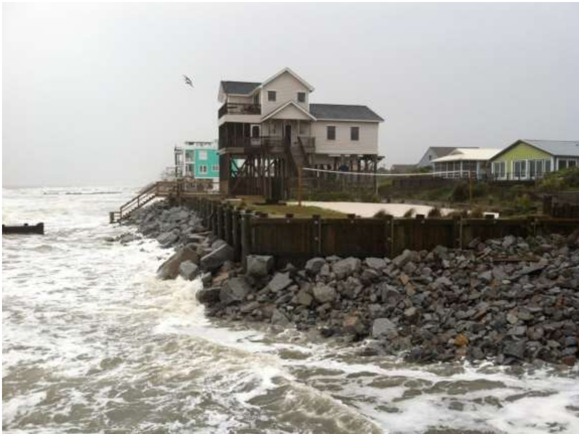
FIGURE 26. EXPOSED SEAWALL AT SUMTER AVE. ALONG THE NORTHEASTERN PORTION OF FOLLY BEACH PRIOR TO THE FEDERAL RENOURISHMENT PROJECT IN 2014.
