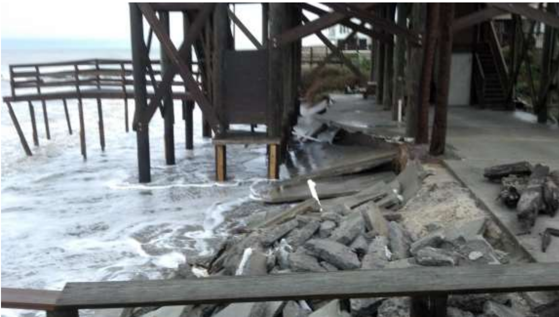
FIGURE 41. PROPERTY DAMAGE ON THE NORTHEAST PORTION OF FOLLY BEACH DUE TO EROSION CAUSED BY HURRICANE SANDY IN 2012.
